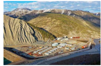
Honey Badger Silver Inc. is advancing the Prairie Creek zinc-silver-lead mine in the western Northwest Territories. The site already benefits from significant previous investment in mine infrastructure.
